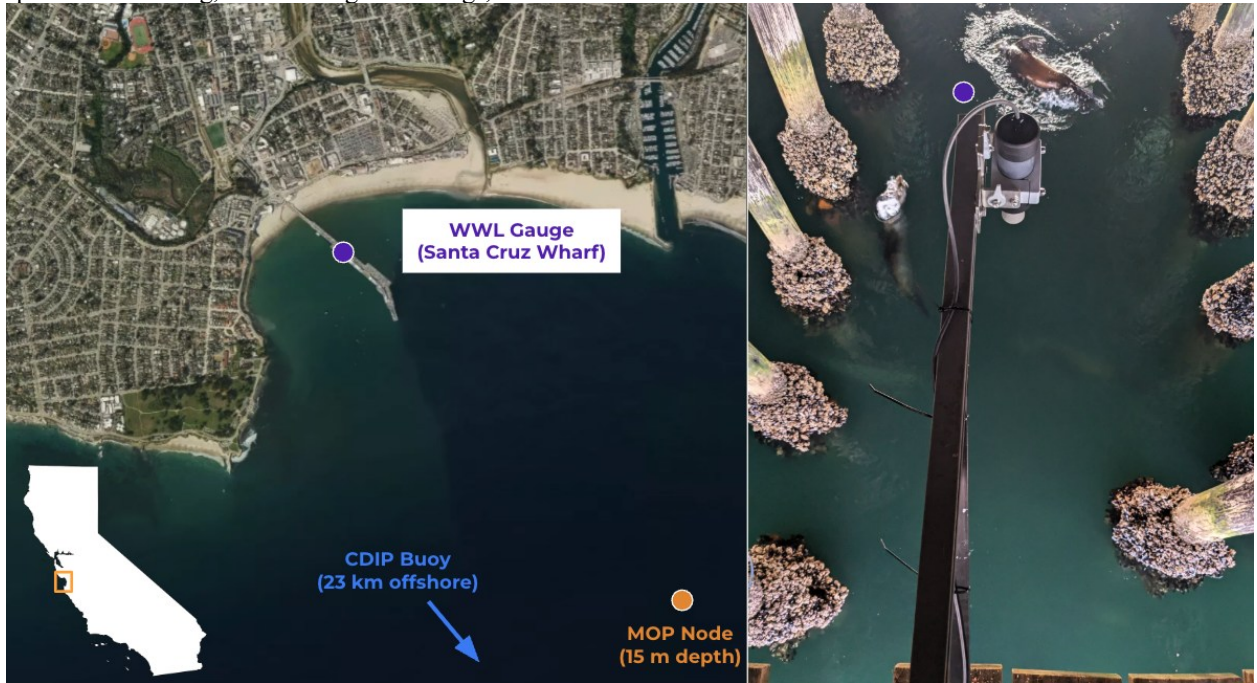
Fig. 1. Left: Map indicating the location of the wave and water level (WWL) gauge relative to the MOP SC-142 model node and the CDIP 156p1 offshore buoy. Right: The installed WWL gauge above the target area underneath the municipal wharf.
