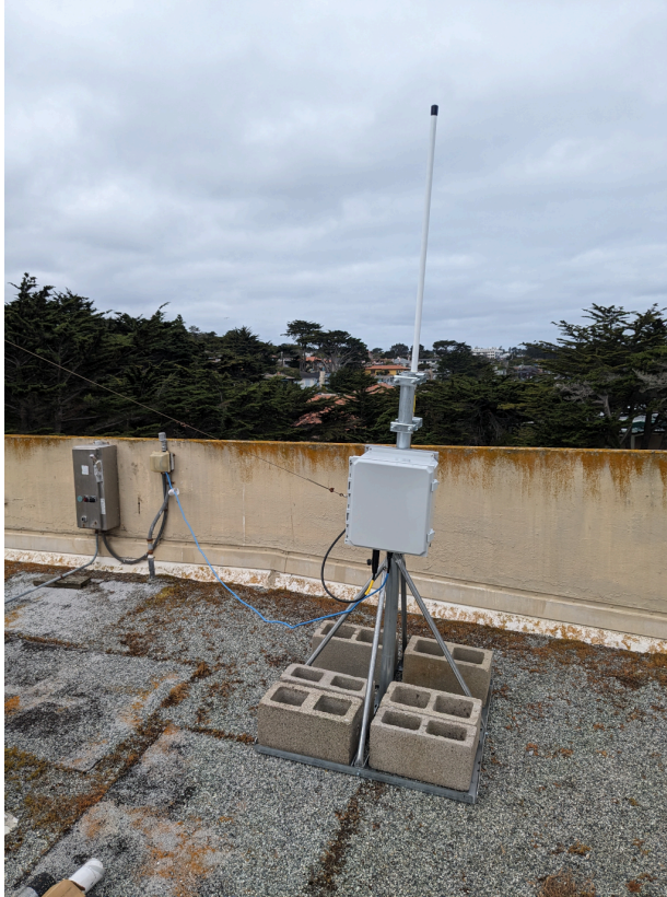
Figure 1: The Luma360 AIS system is shown as mounted to a non-penetrating antenna roof mount system which is portable and easily installed for short term deployments.
